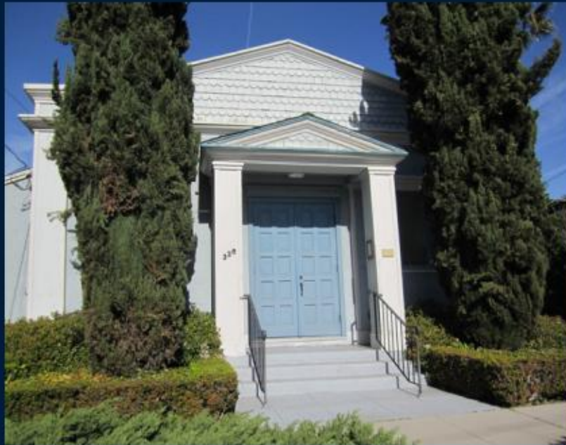
Entrance of the building of Santa Barbara Lodge
